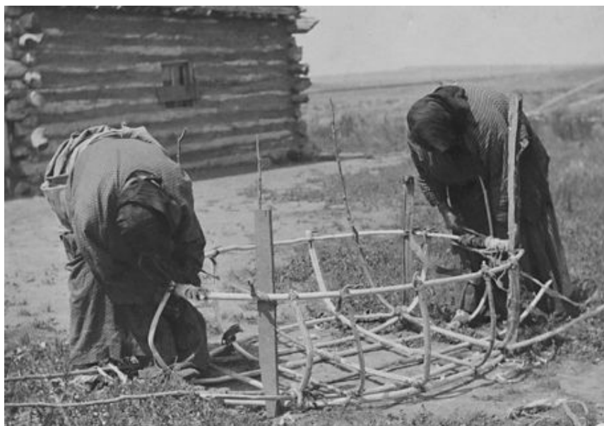
Constructing a Single
